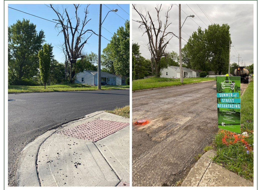
Street Resurfacing. Source: City of Kansas City, MO
