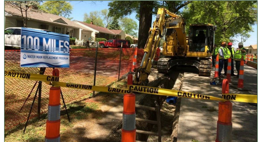
100 miles of water main replacement. Source: Kansas City Star
