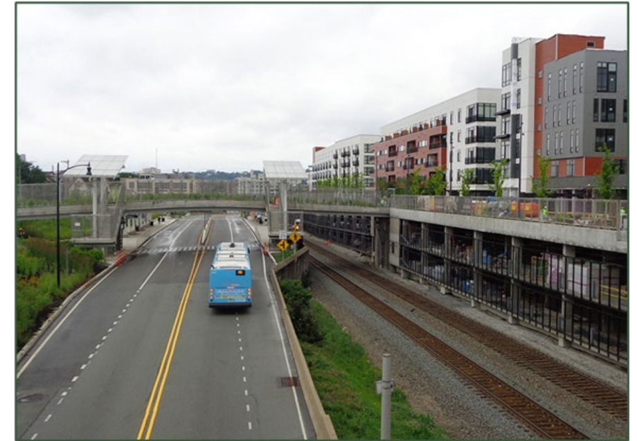
East Liberty Busway Station, Pittsburgh, PA
