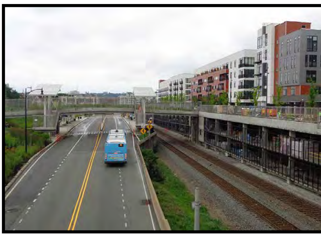
East Liberty Busway Station, Pittsburgh, PA
