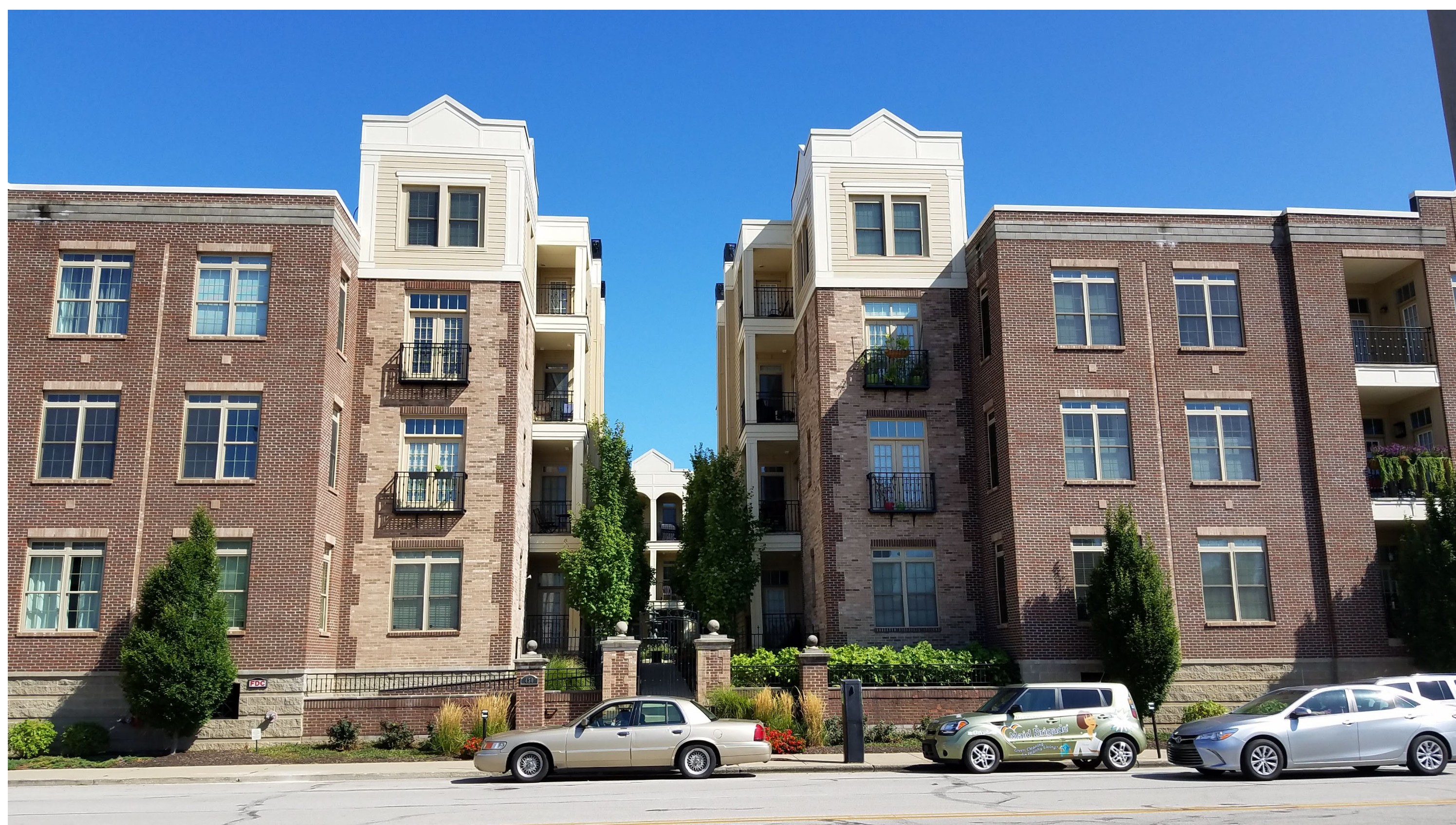
Large Courtyard Apartment Building
